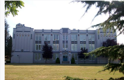
Front of Building
